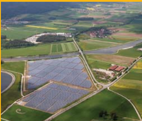
Bavaria Solar Park - 10 MW - Bavaria, Germany
