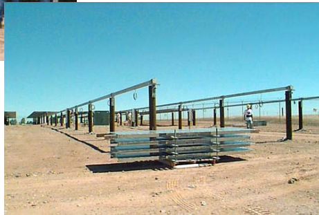
Pile Driven Support Columns
