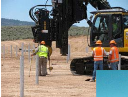
Pile Driven Support Columns
